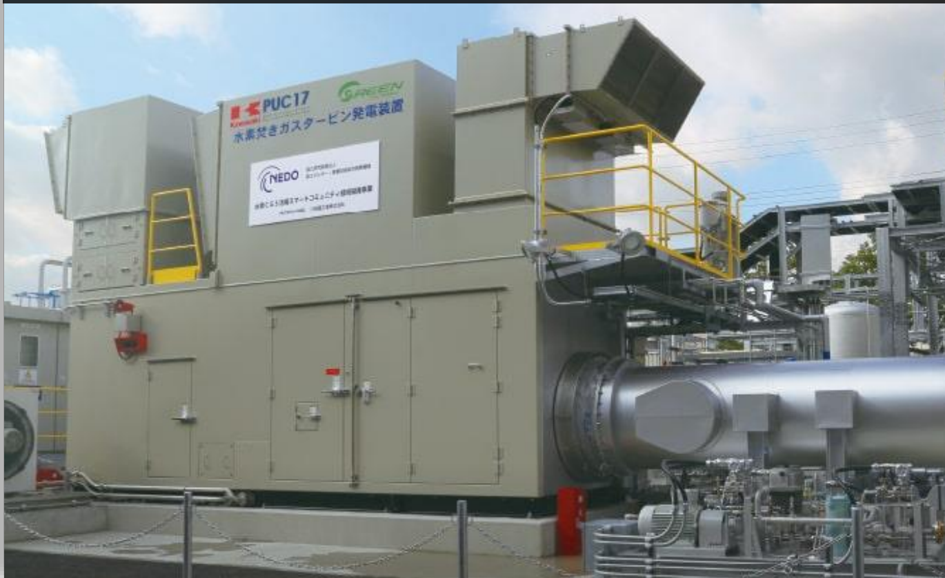
Hydrogen Co-Generation System
