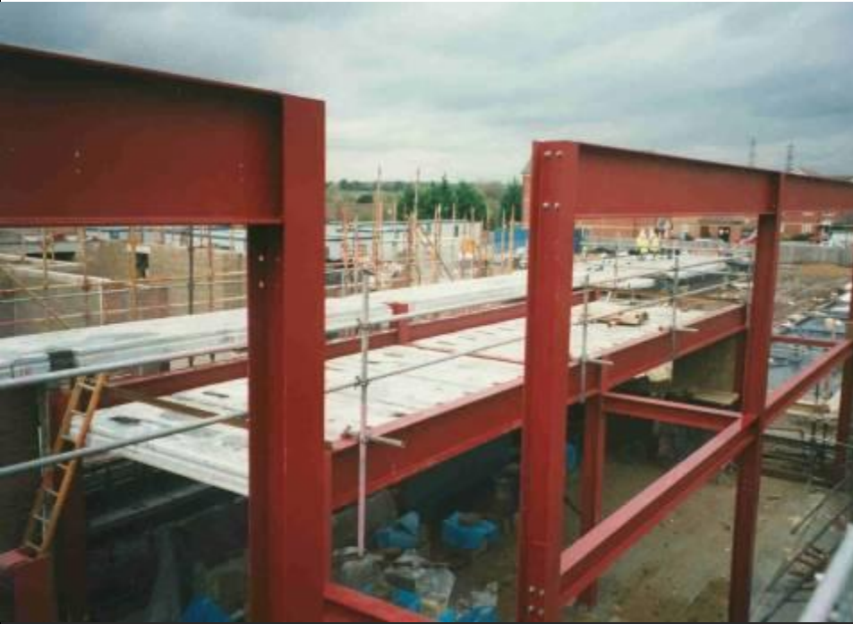
Reclaimed steel -previously used for station work in Brighton
