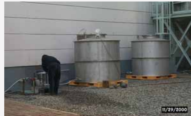
DBA Supplying System
