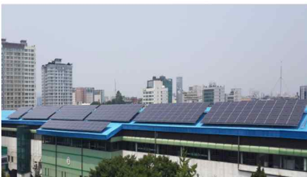
[ Guui Station, 100kW, Completion '13.6.30 ]
