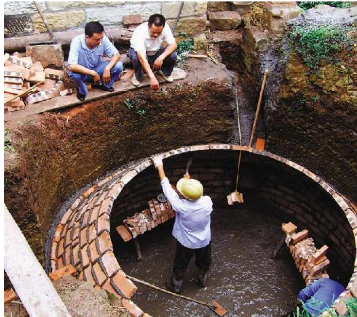
Rural household biogas construction
