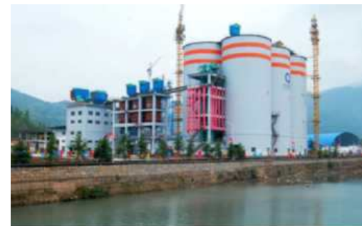
Waste heat power generation of Conch Cement Co., Ltd.
