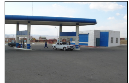
Petrol station /fuel/ area
